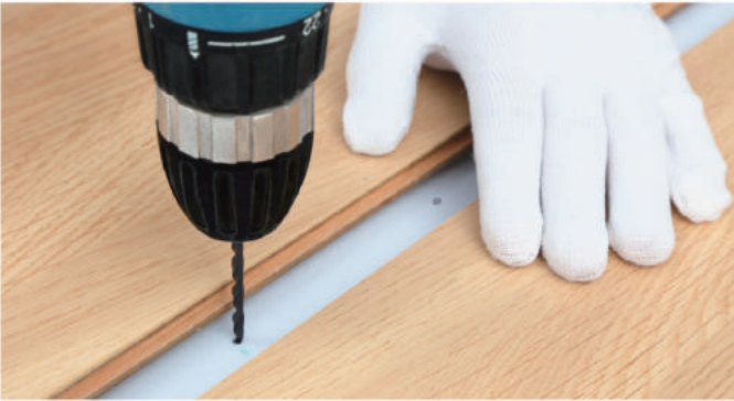
1. Hole positioning & drilling 孔定位并钻孔
