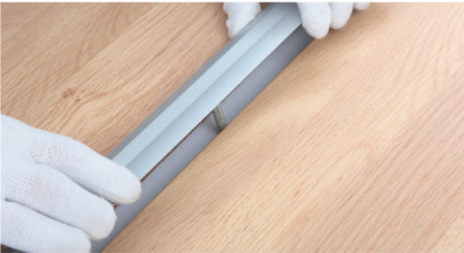
3. Position screws over hole 螺丝定位
